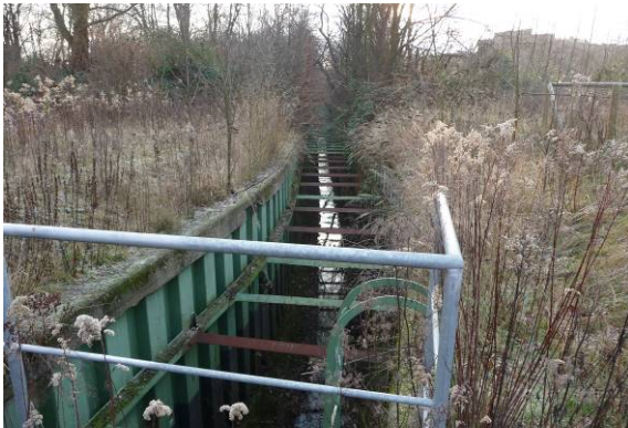
massiver Verbau: Spundwand
