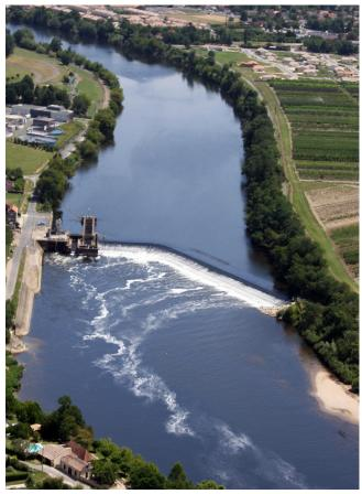
Although the three dams on the river Dordogne in Tuilières (upper left), Mauzac (lower left) and Bergerac (right) are equipped with fish ways, only a minor part of the allis shad population is able to pass the dams. The same applies to the dam at Golfech on the Garonne river.
